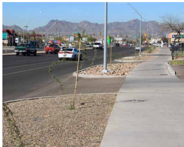
Wide sidewalks installed on newly improved urban arterial roadway. A 12-foot landscaping strip, continuous level 8-foot sidewalks, 11-foot travel lanes, and future tree growth in the planting strip make this a high-quality arterial pedestrian facility.
