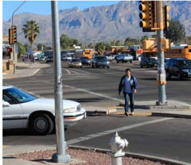
“Porkchops” can reduce crossing distances, but vehicles may pull into crosswalks if not highly visible with signs
