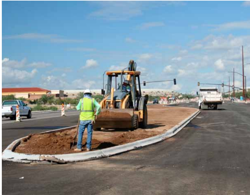
Building a raised median as part of the La Cañada improvement project.
